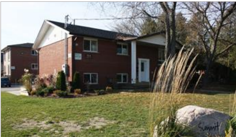
78 Stanley Avenue - Kitchener ON N2K 2B2
